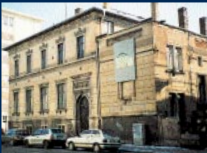
Building previous to renovation Gustaf-Adolf-Straße
