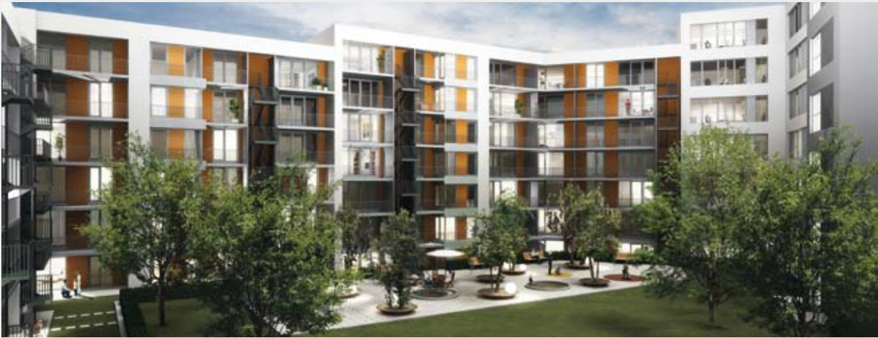
Stuttgart "Südtor" – View of courtyard
